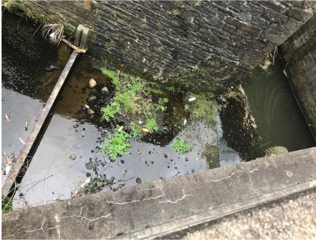
Figure 9 – View of exit of channel feeding the Tennant Canal and removable control weir.
