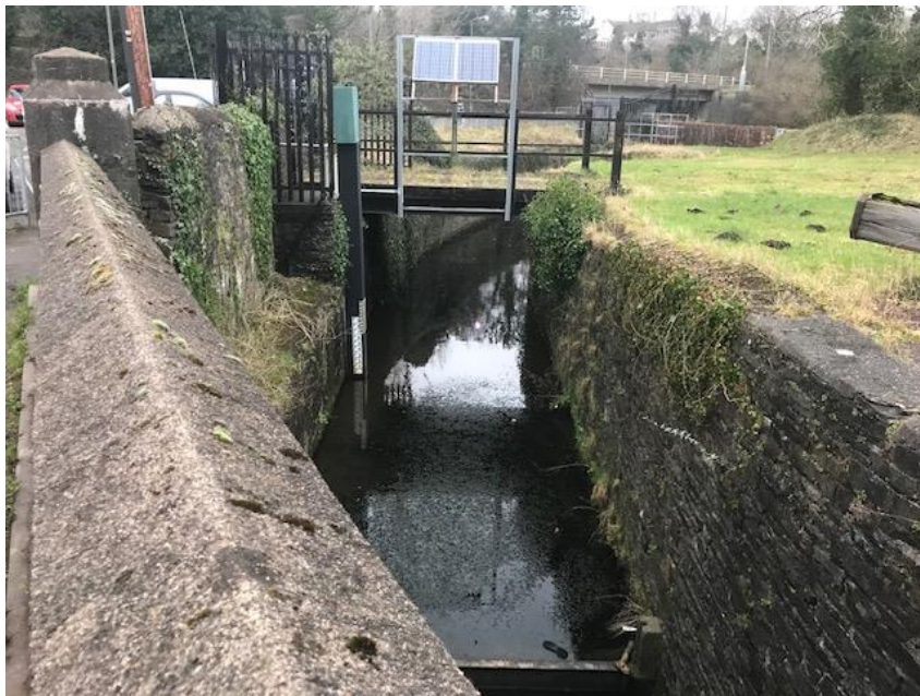
Fig 1 - Tennant Canal Feeder Channel.
