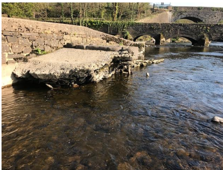
Figure 4 - View of remaining weir alongside the fish pass.
