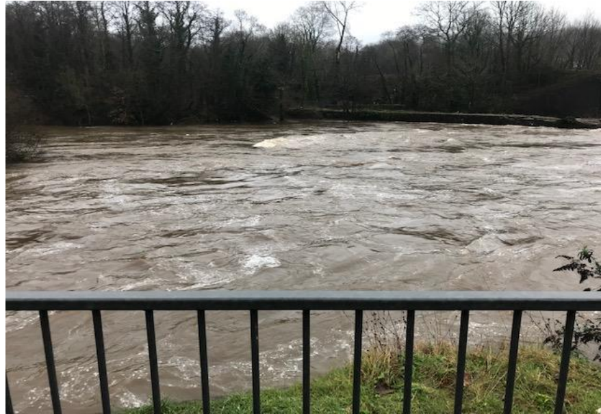
Figure 6 - View across weir from Eastern back illustrating negligible hydraulic impact of current arrangement in partial flood conditions.
